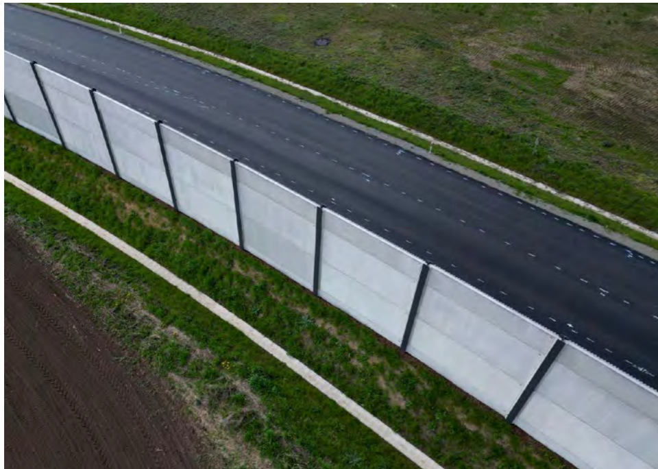
Figure 17. Noise Barrier Wall
